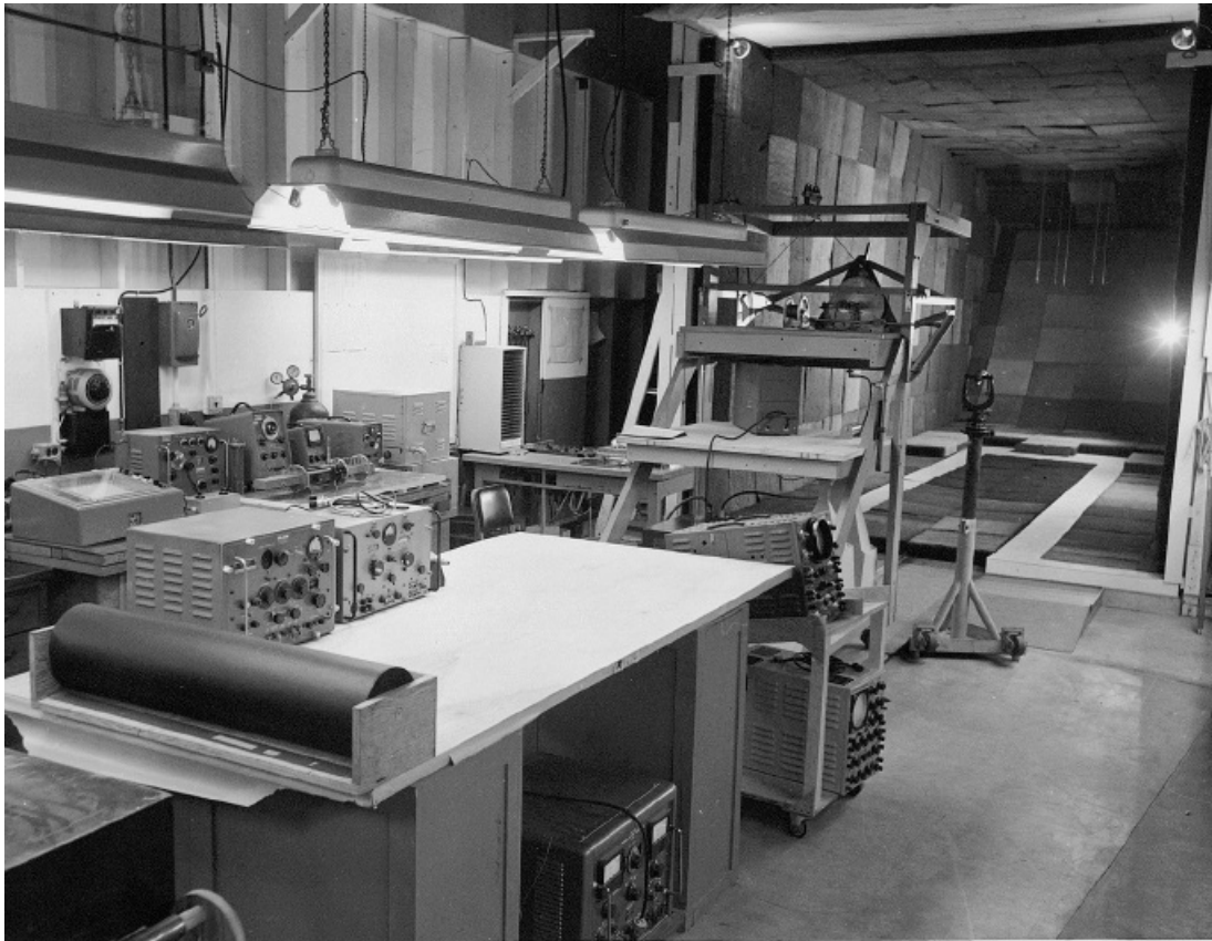
A rare look at Building 82, inside the fabled Lockheed Skunk Works, circa 1957. The world's first anechoic chamber can be seen at the far rear of the room. Shoe-sized models of the CIA's spy planes would be hung from the ceiling and tested. ( Collection of Lockheed Martin )
