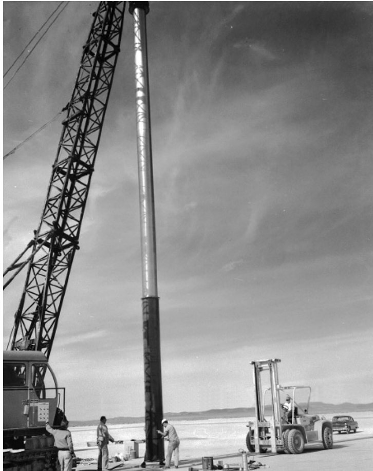
Setting up the legendary Area 51 pylon, or radar test pole. The radar antennas, manned and monitored by EG&G, were located a mile away from the pole. ( Collection of Roadrunners Internationale/CIA )
